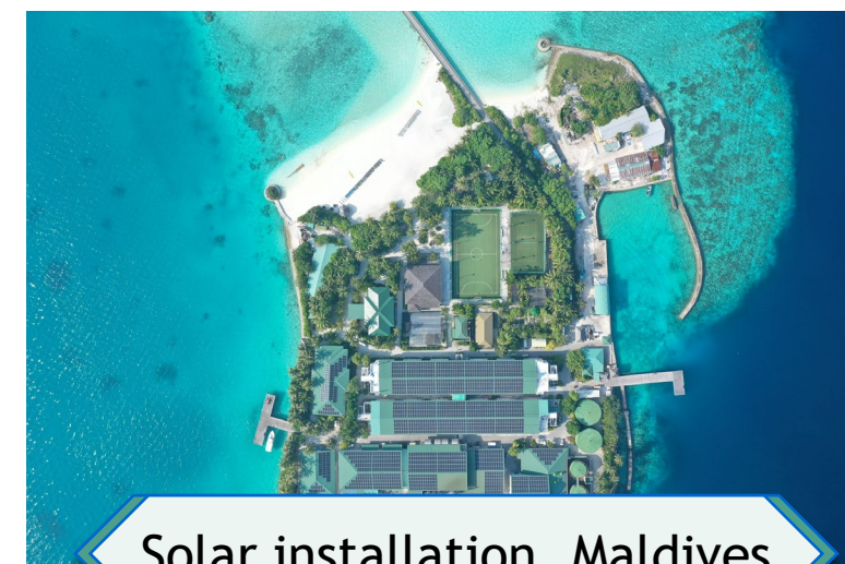
Solar installation, Maldives
